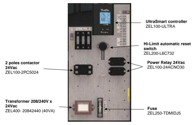
Figure 16: Electrical panel - Combomax Ultra 7,5 & 9 kW
