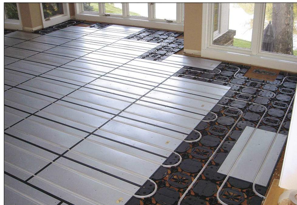
Simple, versatile, cost-effective radiant heating. VersaTherm's surface is highly conductive for exceptionally even temperature distribution and high heat output.
