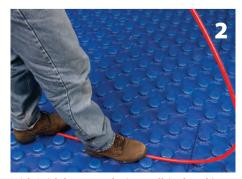
With Quicktherm panels, just walk in the tubing and reduce installation time by up to 75%!
