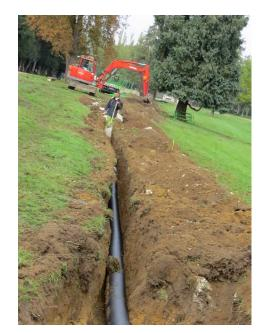
Up to a trench depth of 4 feet, we recommend digging a vertical trench; deeper than 4 feet, we recommend a V-shaped trench.
