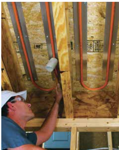
You can install RadiantPEX-AL on the underside of a subfloor, using underfloor plates.
