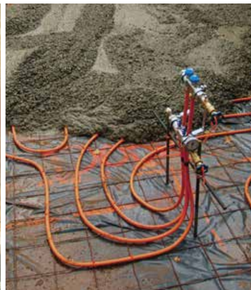
RadiantPEX-AL stays where you want it, making tie-down easier.
