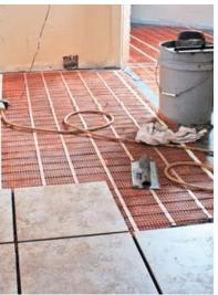
Roll out mat and secure to the floor. Trowel thin-set and lay tile.
