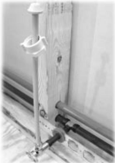
WaterPEX riser, 1/4-turn CrimpRing x compression stop, and PEX stubout bracket.
