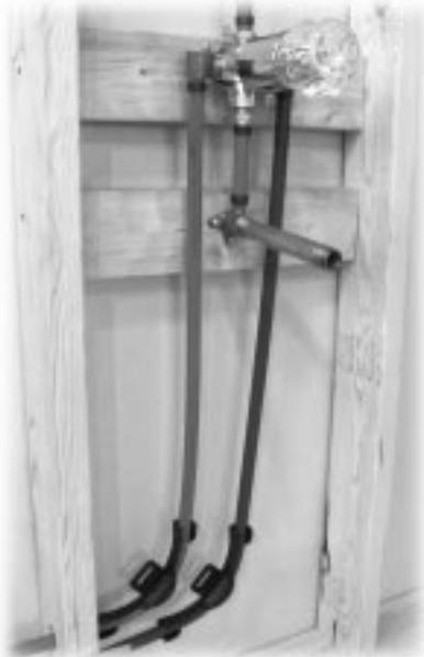
Rough-in at shower using adapters, elbows, drop ear elbow, and bend supports.
