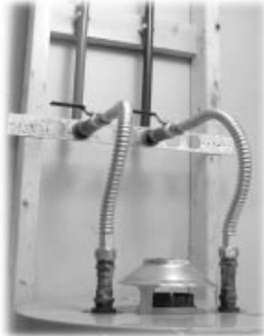
Corrugated supply lines, full-port shut-off valves, SnapClips, and stubout bracket.
