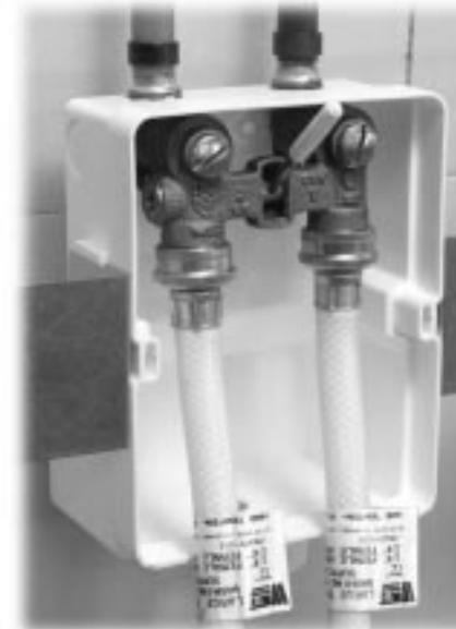
Single-lever WaterOff Washing Machine Control Center with 1/2" CrimpRing fittings and flexible PVC supply lines.
