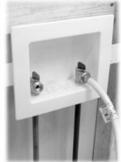
Dual-valve washing machine enclosure with 1/2" CrimpRing fittings and flexible PVC supply lines.
