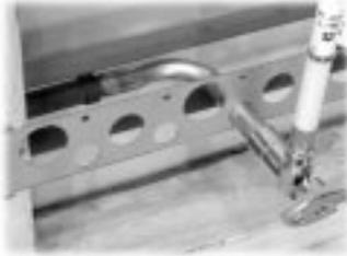
WaterPEX 1/4-turn stop, PVC riser, and copper stubout with bracket.
