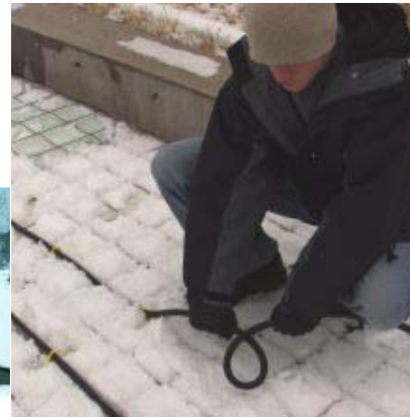
Onix is just as flexible in cold weather as in hot, so you can install it year-round.
