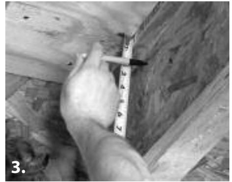
3. Measure 2" below the subfloor and mark the joists on both sides of the joist cavity.
