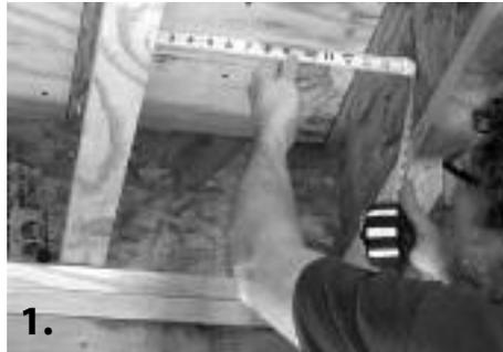
1. Measure between the floor joists where mat(s) will be installed. Measure the width of the mat selected to fit between these joists. The difference between these measurements determine how much mat mesh remains for stapling to each side of the joists. Because the distance between floor joists can vary, taking these measurements will help ensure the mat will be centered between the joists. It is also prudent to test fit the mat by holding the mat up into the joist cavity.
