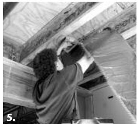
5. Hold the mat up along one joist and begin stapling the mat mesh along the 2" mark from the subfloor. Staple every 4" to 6" for about 2 ft. to get started.
