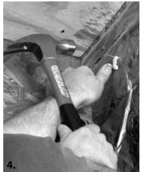
4. To help hold up the power leads while installing the mat, fasten one NailTite over the power leads
