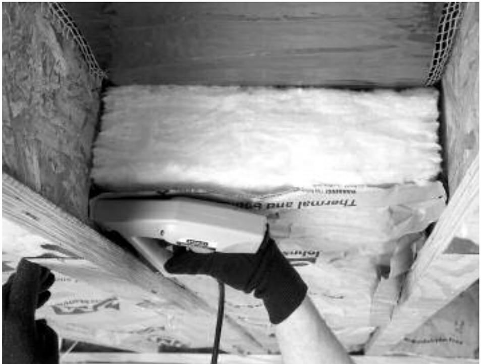
**REMEMBER:** Proper insulating and sealing of the floor cavity is necessary for the performance of HeatWeave UnderFloor mats.
