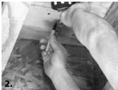
2. If the mat begins near the rim joist, measure about 6" out from that rim joist. This will allow enough room for the mat power leads, and will prevent unnecessary heating of the wall cavity above the floor.
